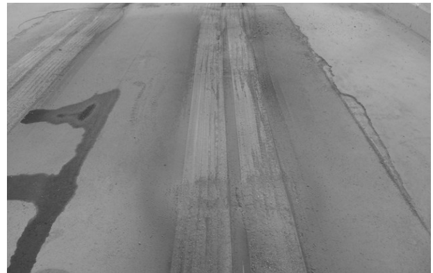
Fig. 12. Surface after Accelerated Pavement Test
