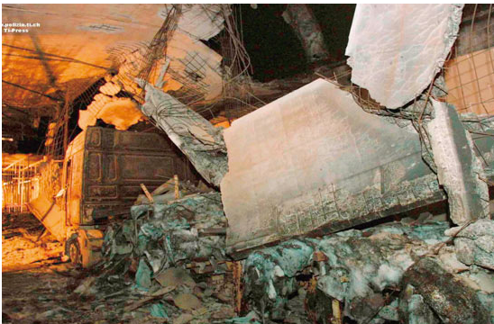
(c) Gotthard Tunnel
