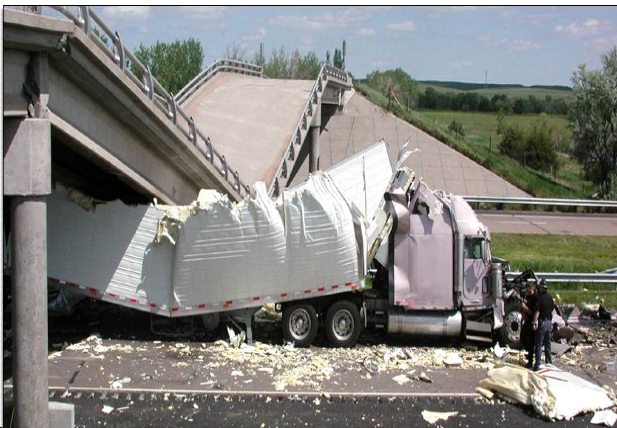
Fig. 1 Bridge collapse due to cargo truck collision ( http://cellar.org/showthread.php?t=3475 )
