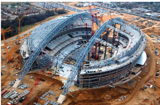
〈Fig. 5〉 Construction method of Cowboys Stadium
