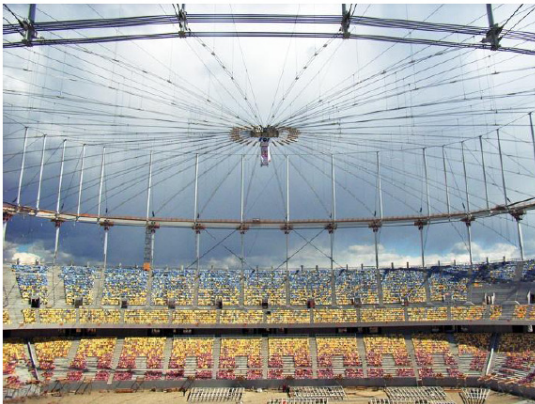
〈Fig. 9〉 The cable net structure in its final position
