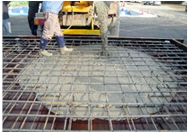
Fig. 7 Construction of Concrete Modular Slab using Self-Compacting Concrete
