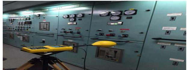
Figure 9: Measurement process of switch board
