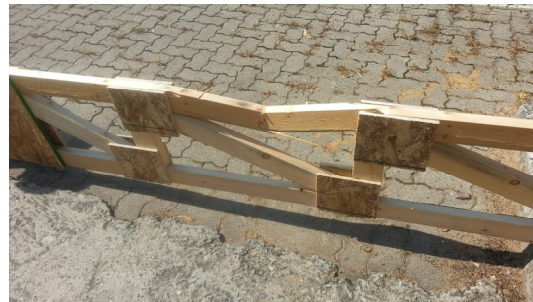
Fig. 10. Failure of upper chord member of flat truss under bending loads.
