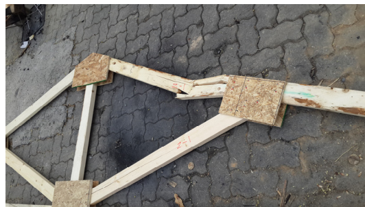
Fig. 8. Failure of upper chord member of roof truss under bending loads.
