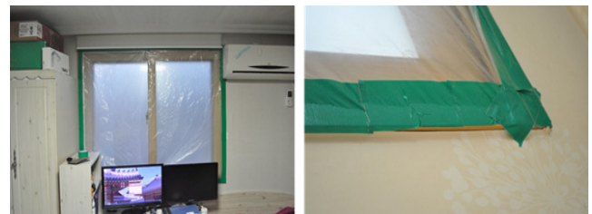
Fig. 2 Sealing of windows
