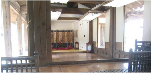
<Figure 3> Lift-open structure door-wall in the room of Yoon Taek-Young, Haepoong Buwongun
