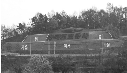
Figure 3. Site I after test construction (cut slope in Seosejong IC).
