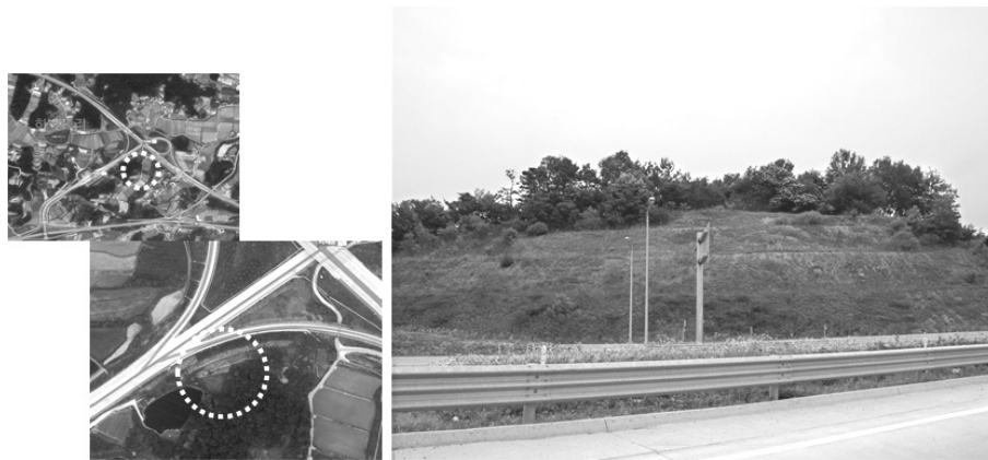
Figure 1. Site I for test construction (cut slope in Seosejong IC).
