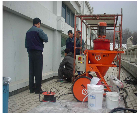
Fig. 7. Sealant injection equipment.
