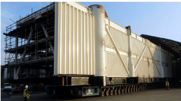
Fig. 1 Typical blast wall on offshore structures (Mech-Tool Korea Inc., 2013)
