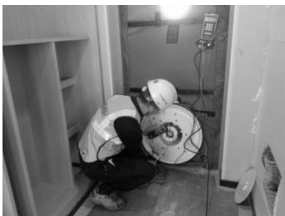
Fig. 2. Door fan leakage-proof measurement
