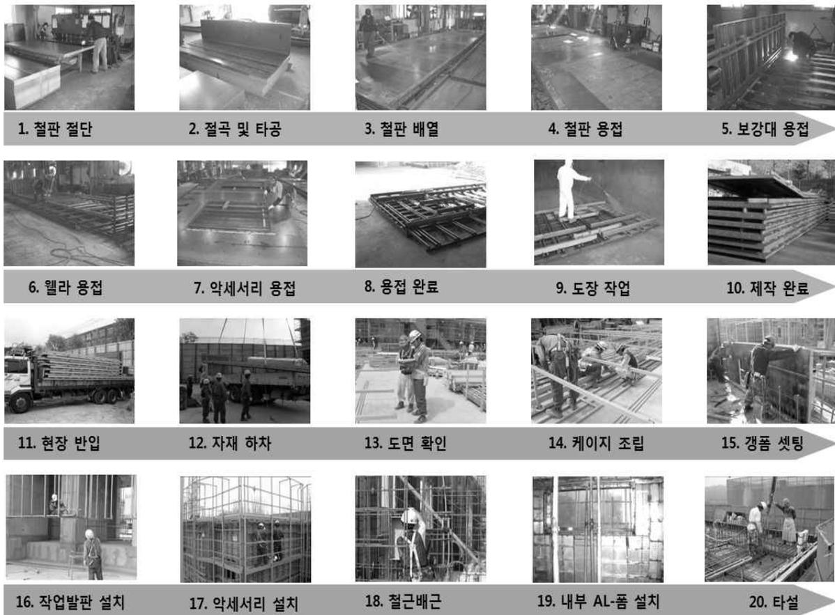
[Figure 1] Gang Form Production And Construction
