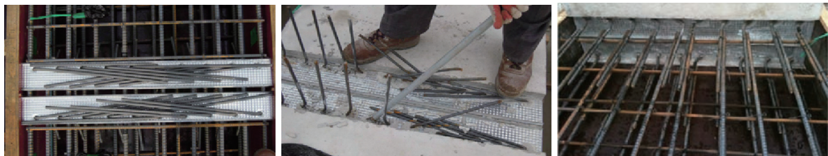
(a) Placing bent re-bars
