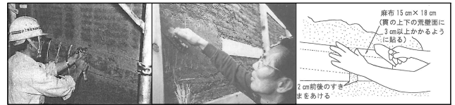
Fig.7 Japan Nukibuse(貫伏せ) techniques(새끼줄, 짚여물, 삼베)
