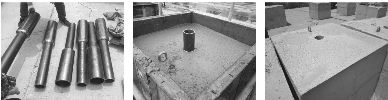
(a) Mold of borehole
