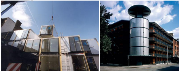
Figure 3. Modular House, Murray Groove, England
