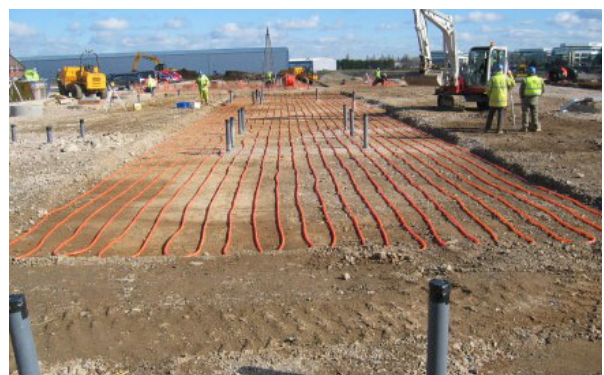
Fig. 13 Construction of the Store Array (ThermalBank) - Beneath the School
