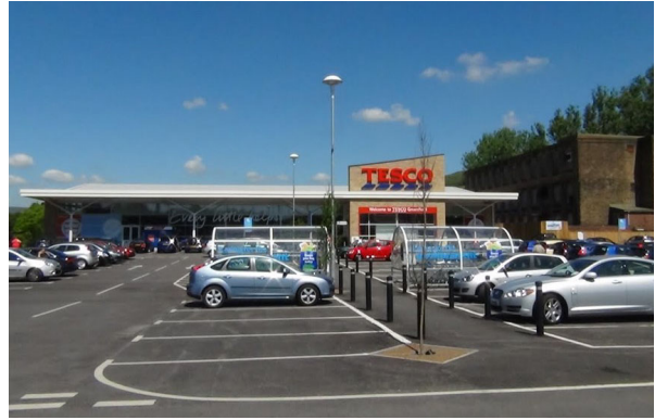
Fig. 14 Tesco Greenfield Supermarket
