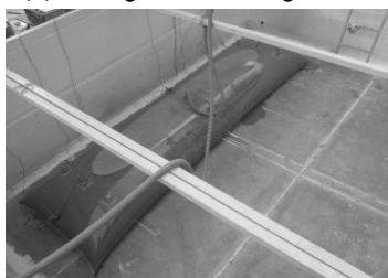
(c) Filling of the Dredged Soil
