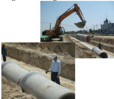
FIGURE IV PIPELINE CONSTRUCTION AND READING
