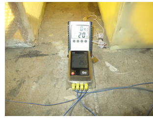
Photo 7 Installation of data logger
