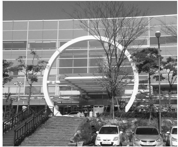
Fig. 1. Erected Example of Horseshoe Arch as an Entrance Portal at the Wonkwang University Hospital
