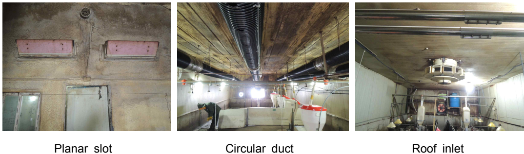
Fig. 4. Inlet ventilation facility using in weaned pig house.
