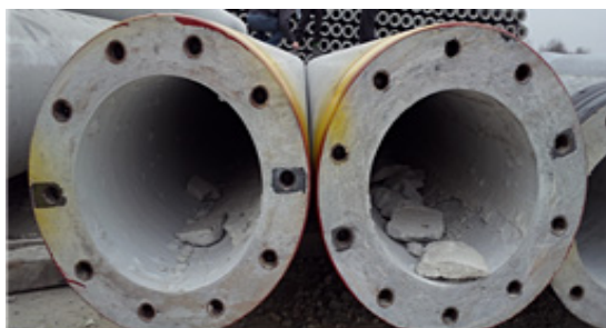
Fig. 9. Inner Side Condition of PHC PILE
