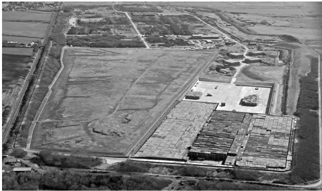
Fig. 1. VLLW Disposal Facility of UK [6].
