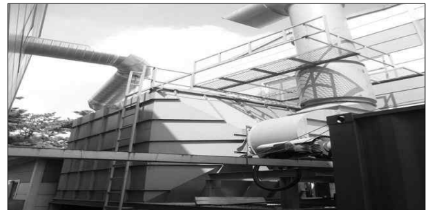
b.Activated carbon adsorption external [Figure 1] Adsorption inside and outside
