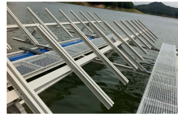
Fig. 5. Previous solar module support frame
