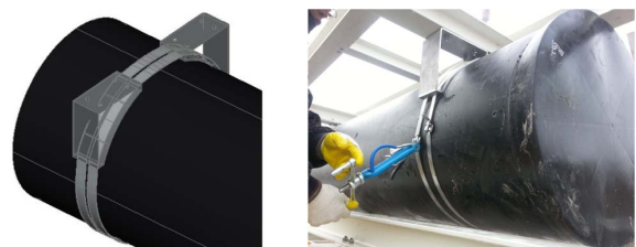
Fig. 7. Floating system using steel bend
