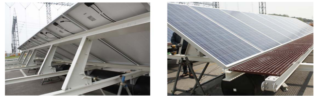
(b) Solar module support and foothold member
