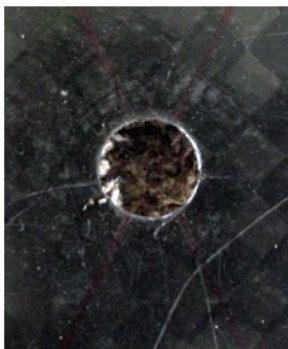
Fig. 8. Removal of damaged area
