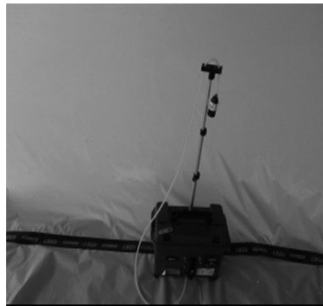
Fig 3.4. Photo for asbestos sampling.
