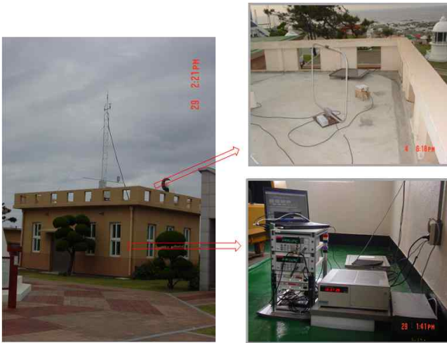
Fig. 7 Management office for maritime navigation aids and dLoran system at the roof and inside of the office
