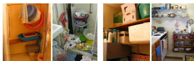
(a) Altering bathroom (b) Installing storage shelves
