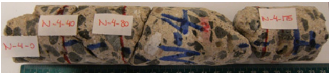
Fig. 4 Sample cored from RC column after fire test
