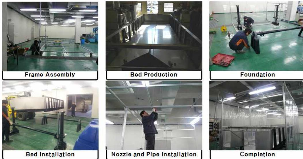
Fig. 2. Installation Process of Rainfall-Runoff Simulator
