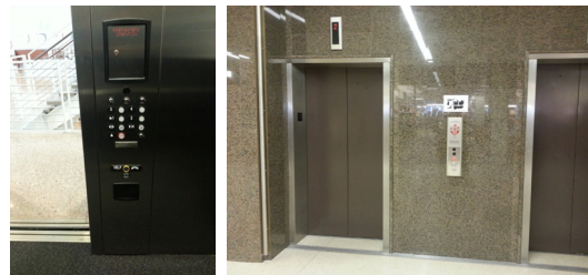
Figure 7. Most lifts provided convenient location of controller for wheelchair users, but no braille sign.(TAMU, UTA)
