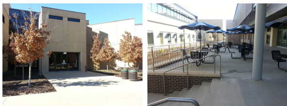
Figure 2. Main entry of every school provided easy access, while some of sub-entry at UH(left) and UTD didn't provide ramp.
