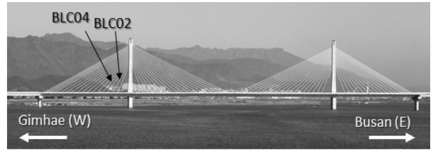
Fig. 4. Hwaryung cable-stayed bridge and test cables
