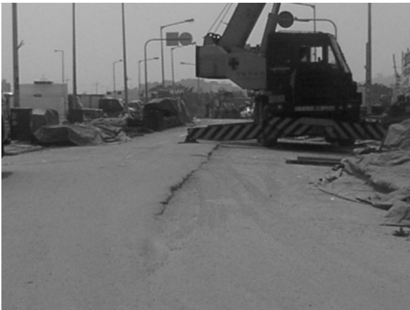
Fig. 2. Road Failure by Excavation
