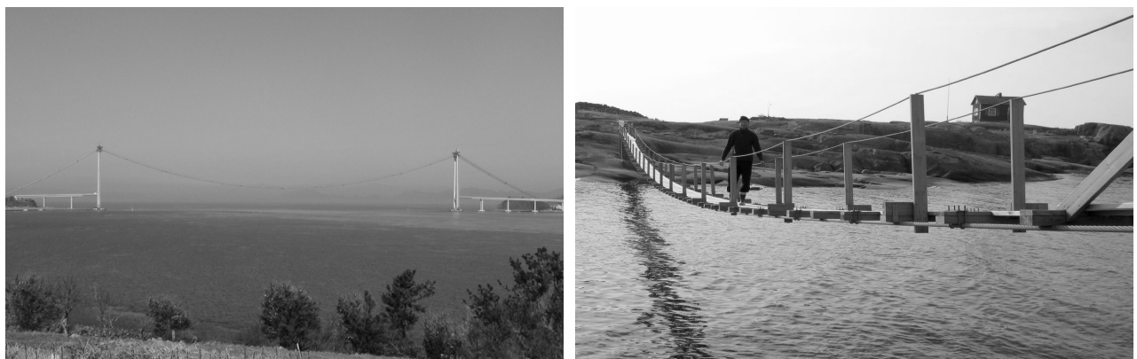
Fig. 3. Catenary Shape Example (from left side Cable of Jeokgeum-Youngnam Bridge, Simply supported Skybridge)
