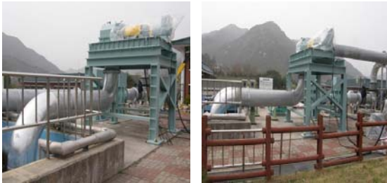
(b) Installation image-A (c) Installation image-B
