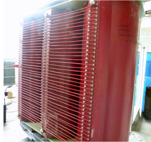
Fig. 3. 1600 kVA, 40 Secondary Transformer
