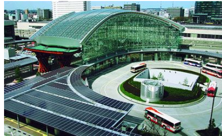
[Fig. 3] Traditional style design of Kanazawa Station (source: Google Image Search of "Kanazawa Station")
