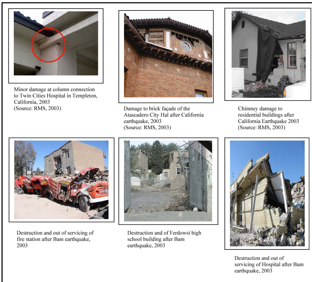
<Figure 2> Comparison of California and Bam buildings destruction in the earthquakes in year 2003
