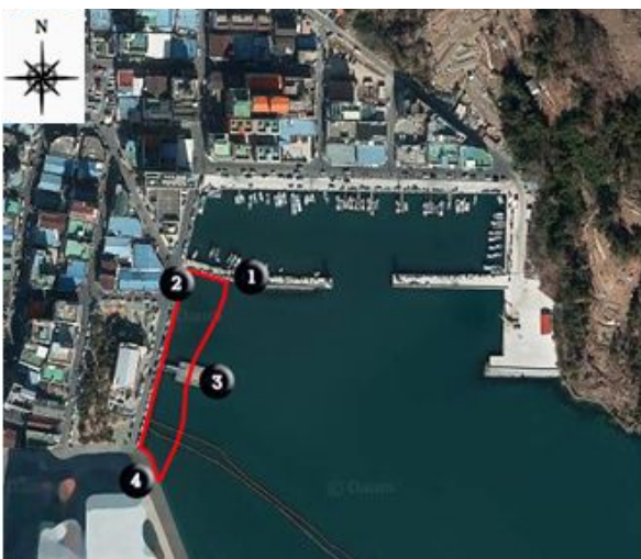
Fig. 9. Waterfront Construction Projects in Ok-po Port.
