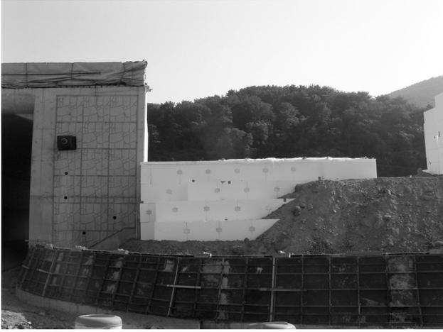
Fig. 11. Construction of EPS backfill
