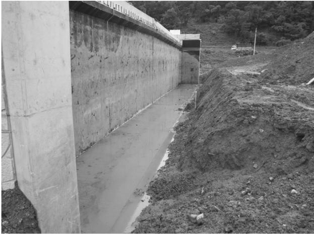
Fig. 8. Excavation of backfill to prevent joint gap
