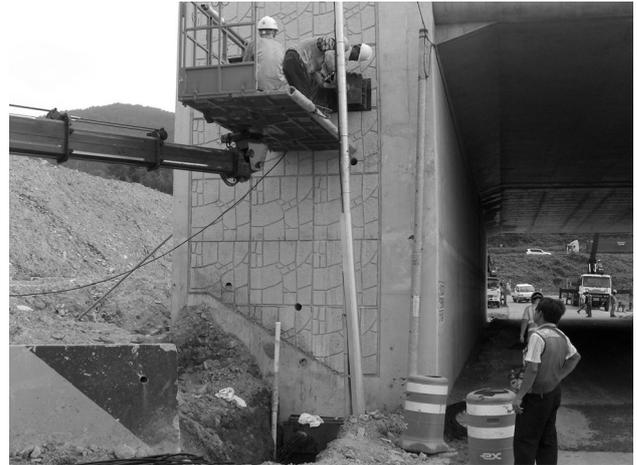
Fig. 9. Installation of pretension rebar to prevent joint gap
