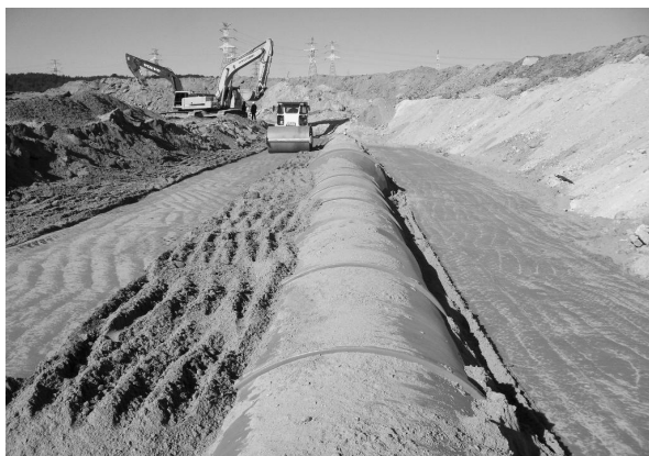
Fig. 2. Construction of GFRP pipe
