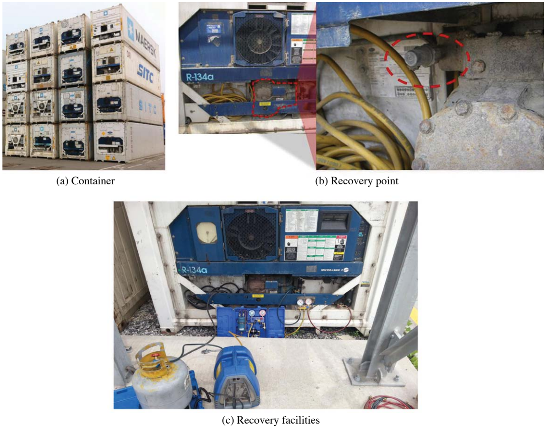
Fig. 2. Pictures for refrigerant recovery facilities of HFC-134a from reefer container.
