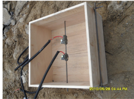
Fig. 4. Shotcrete stressmeters installed in the unstressed mold.
