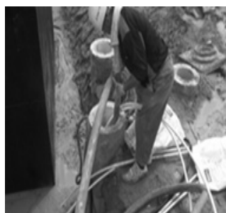
(b) Cement grouting
