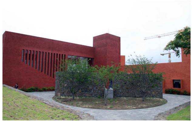
Figure 1. The Gallery of Casa del Agua (front view)
