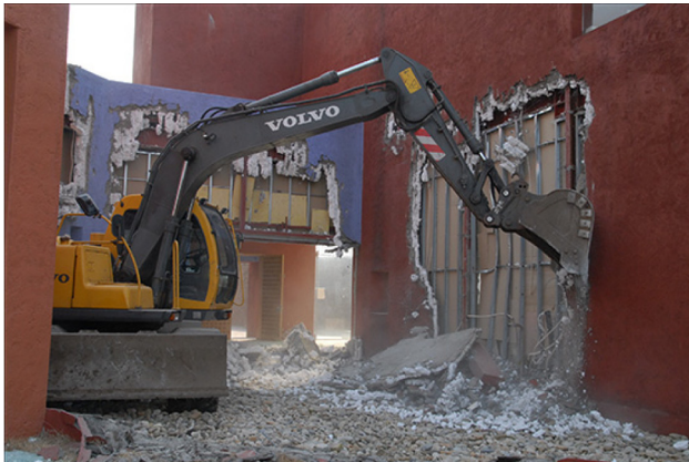
Figure 2. The Gallery of Casa del Agua is Demolished
