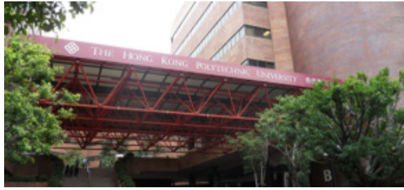
(a) Double layer system (The Hong Kong Polytechnic University, Hong Kong)
